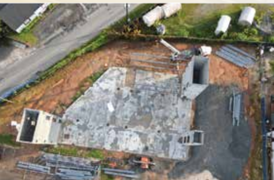
Foundation poured and stairwells in place.
