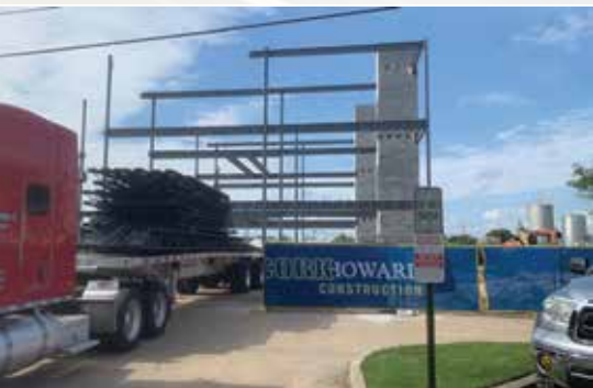
Steel is delivered.
