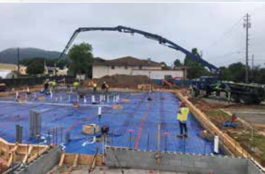
Laying the foundation.
